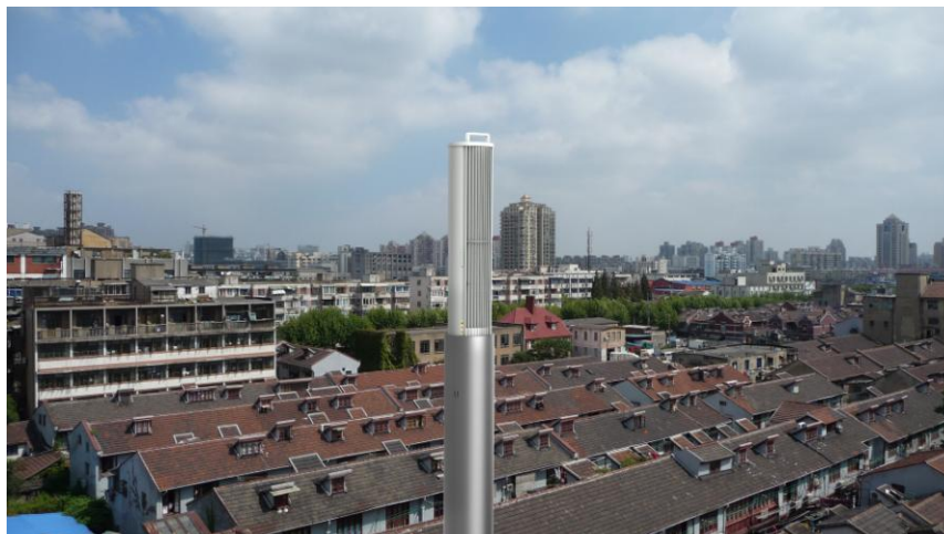
Figure 1-2 AAU3940 modules installed on the top of a building
