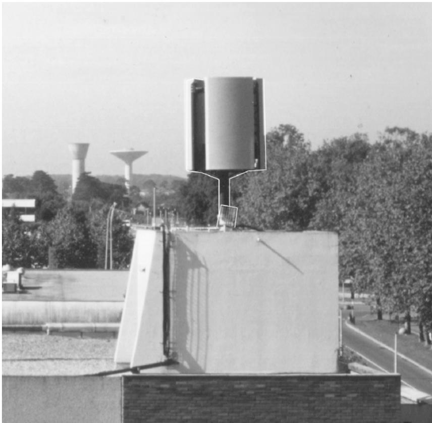
**Figure 3-41 S4000 Smart BTS: Antenna integrated facets**
