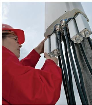
After feederline installation, the optional remote control units (RCUs) can be mounted.
